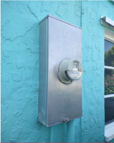
SHOWING MAIN ELECTRICAL SERVICE METER.
