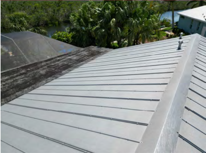
SHOWING CLOSEUP OF THE ROOF RIDGE CAP AND FASTENERS.
