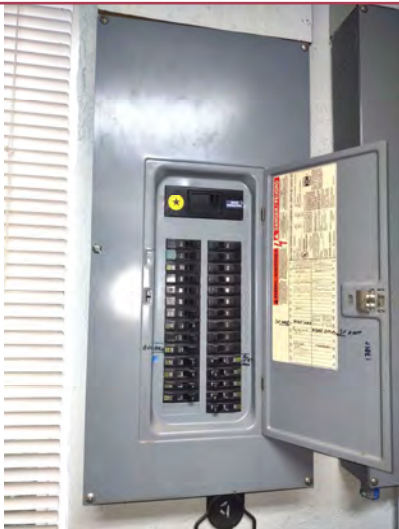
SHOWING 100 AMP MAIN ELECTRICAL PANEL WITH COVER OPEN AND LABELING PRESENT.
