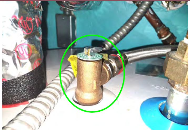
SHOWING WATER HEATER TPR VALVE IS PRESENT.
