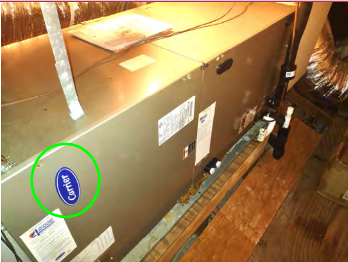
SHOWING CARRIER AC AIR HANDLER UNIT LOCATION IN THE ATTIC.
