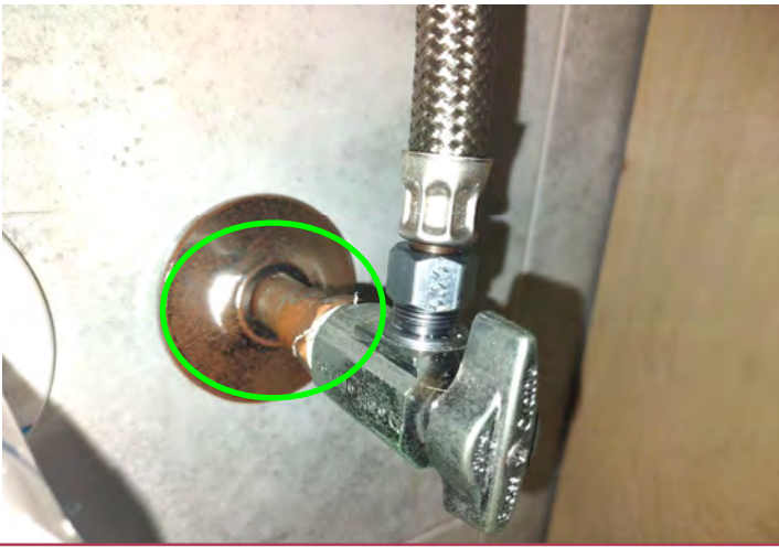
SHOWING DOWNSTAIRS BATHROOM 2 UNDER THE SINK WITH COPPER SUPPLY PIPING PRESENT.
