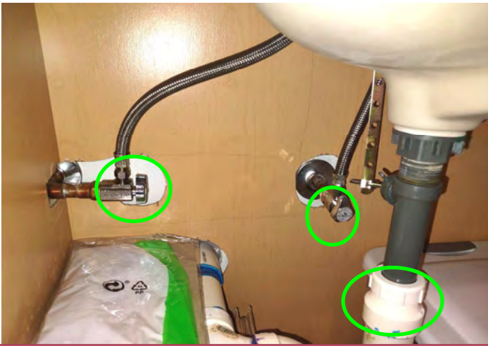
SHOWING DOWNSTAIRS BATHROOM 1 UNDER RIGHT SIDE OF THE SINK QUICK SHUT OFF VALVES PRESENT AND PVC DRAINAGE PIPING.
