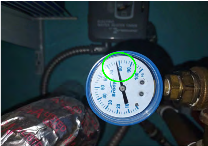
SHOWING ADEQUATE WATER PRESSURE 78 PSI. 30-80 IS ACCEPTABLE.
