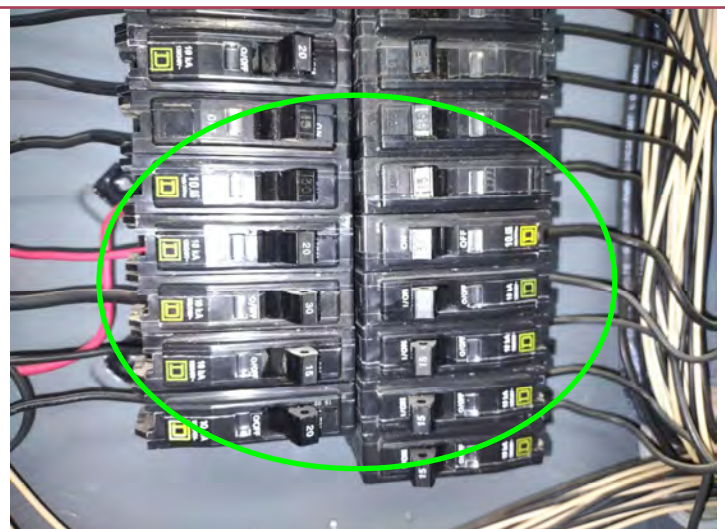
SHOWING 100 AMP MAIN ELECTRICAL PANEL WITH CLOSEUP OF THE CIRCUIT BREAKERS. SHOWING CIRCUIT BREAKERS BRAND SQUARE D.
