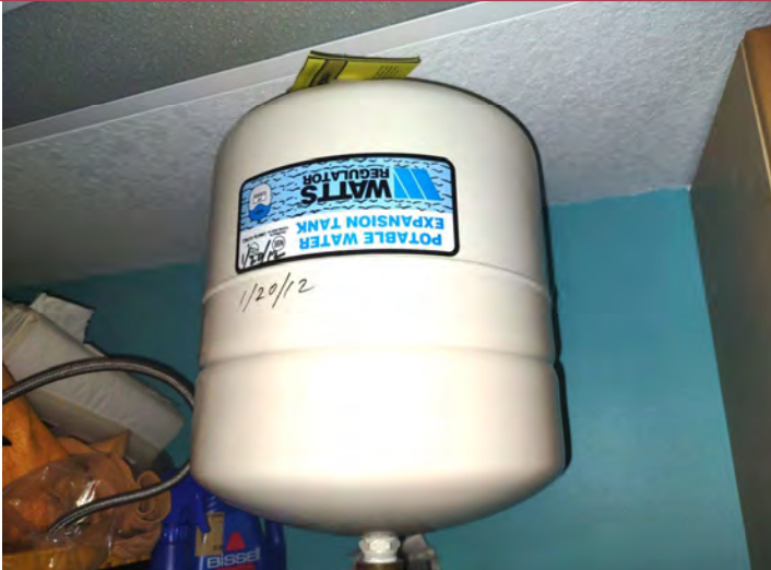
SHOWING WATER HEATER EXPANSION TANK.
