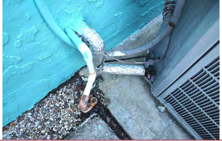
SHOWING AC LIQUID AND SUCTION LINES AND CONDENSATE LINE WITH ADEQUATE DRAINAGE.
