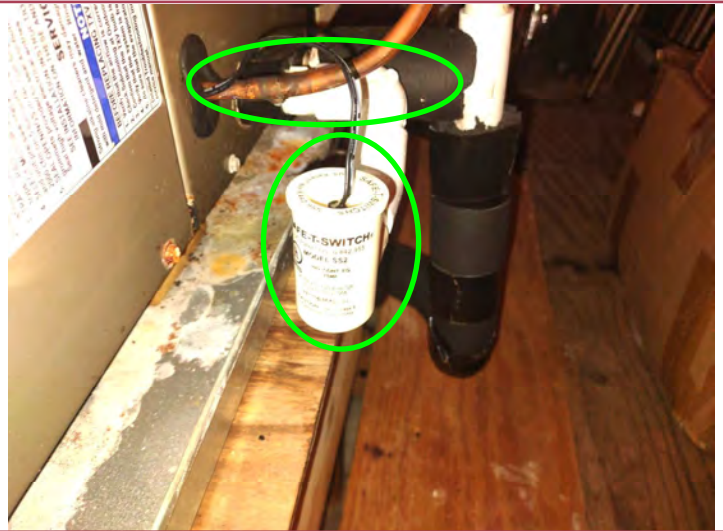
SHOWING AC AIR HANDLER LIQUID AND SUCTION LINES AND AIR HANDLER OVERFLOW SHUT OFF SWITCH. NO LEAKS AT THE TIME OF THE INSPECTION.
