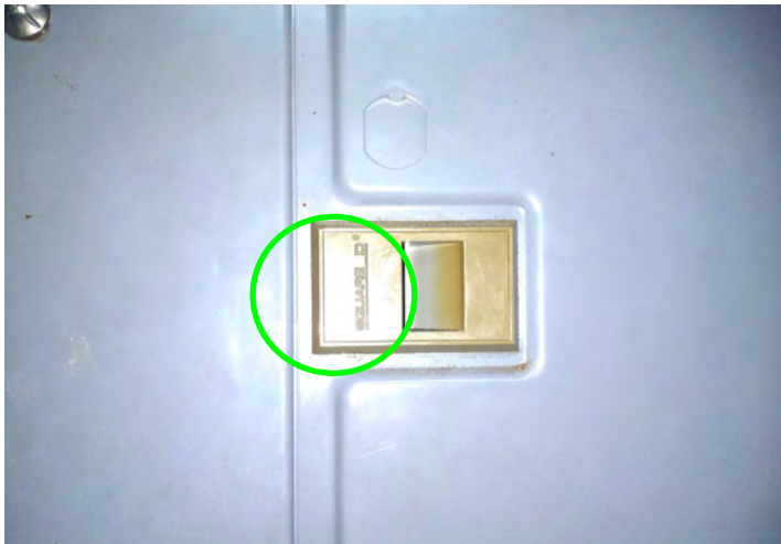
SHOWING 200 AMP MAIN ELECTRICAL PANEL BRAND IS A SQUARE D.
