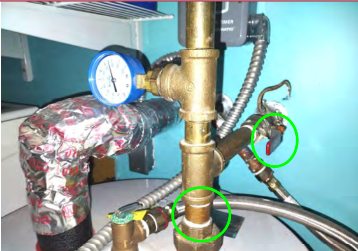
SHOWING WATER HEATER COPPER SUPPLY PIPING AND SHUT OFF VALVE ARE PRESENT.
