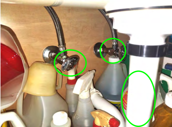
SHOWING UNDER LAUNDRY ROOM SINK QUICK SHUT OFF VALVES PRESENT AND PVC DRAINAGE PIPING.
