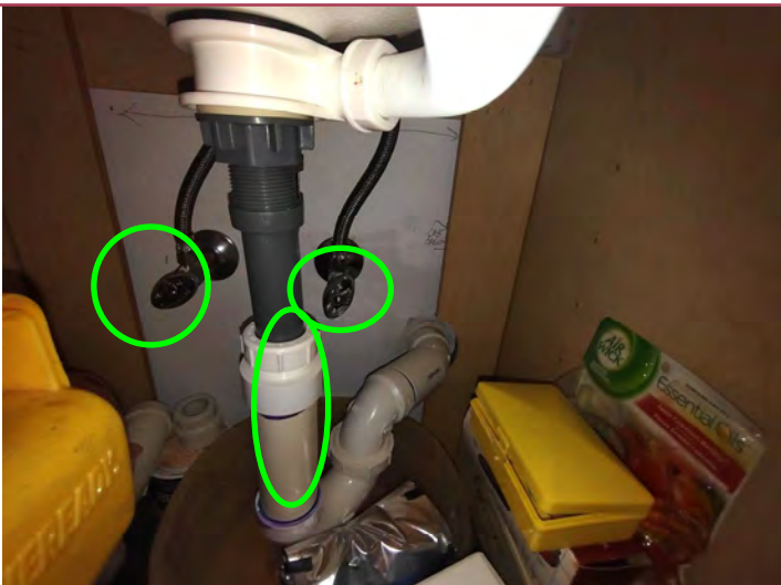
SHOWING UPSTAIRS BATHROOM LEFT SIDE UNDER THE SINK WITH QUICK SHUT OFF VALVES AND PVC DRAINAGE PIPING.
