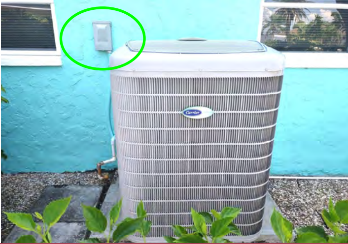
SHOWING AC COMPRESSOR WITH A PROPERLY LOCATED DISCONNECT.
