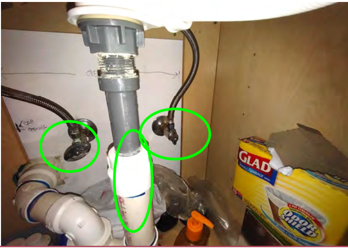
SHOWING UPSTAIRS BATHROOM UNDER THE RIGHT SIDE OF THE SINK WITH QUICK SHUT OFF VALVES AND PVC DRAINAGE PIPING.
