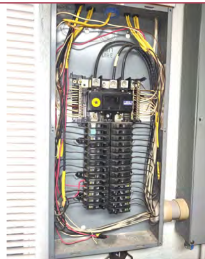
SHOWING 100 AMP MAIN ELECTRICAL PANEL WITH COVER OFF.
