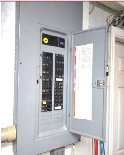
SHOWING 200 AMP MAIN PANEL WITH COVER OPEN AND LABELING PRESENT.
