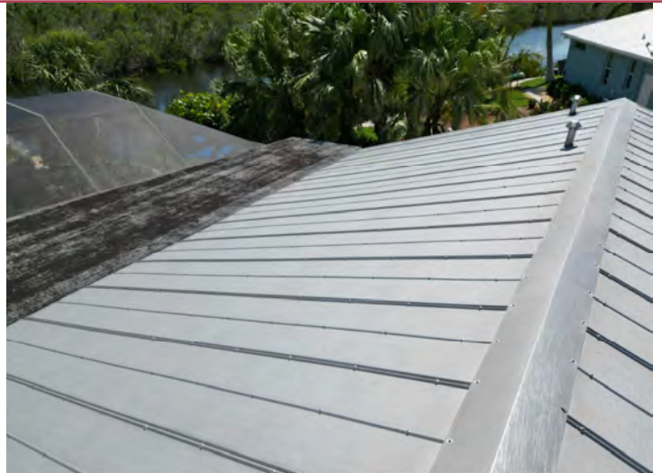
SHOWING CLOSEUP OF THE RIDGE CAP AND FASTENERS.
